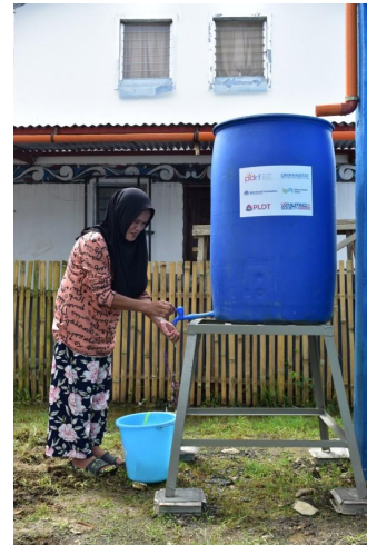
A resident of Hadiya village trying the new rainwater catchment system
